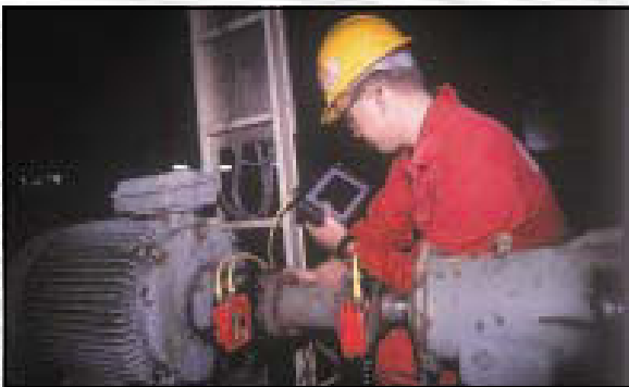
Shaft alignment of motor and pump using Fixturlaser Shaft 200 .
